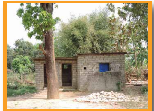
This sanitation facility is shared amongst 550 students and staff.
